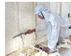
fig.18 削り作業
